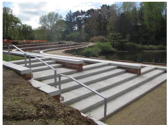
Figure 12: The Alexander Steps, a major project in 2011
